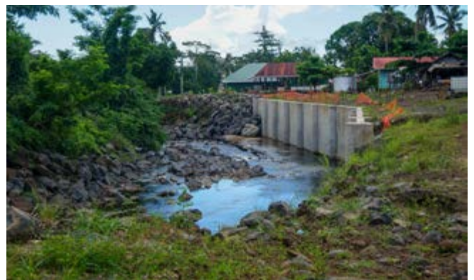
Flood protection near Malia’s home. The Green Climate Fund is supporting work to benefit 27,000 people living in the flood-prone Vaisigano river catchment in Apia, Samoa.
